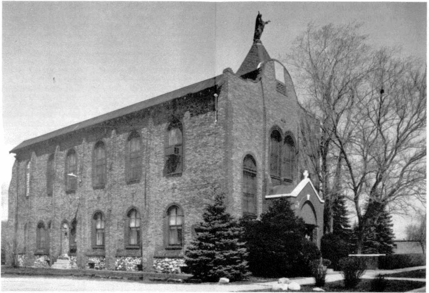
In 1902, parishioners enclosed the church with bricks made in the nearby Purington Brickyard, which altered the style of the building. The arched windows and large curved gable over the entrance are reminiscent of the Mission style of architecture. (Bob Thall, photographer)
